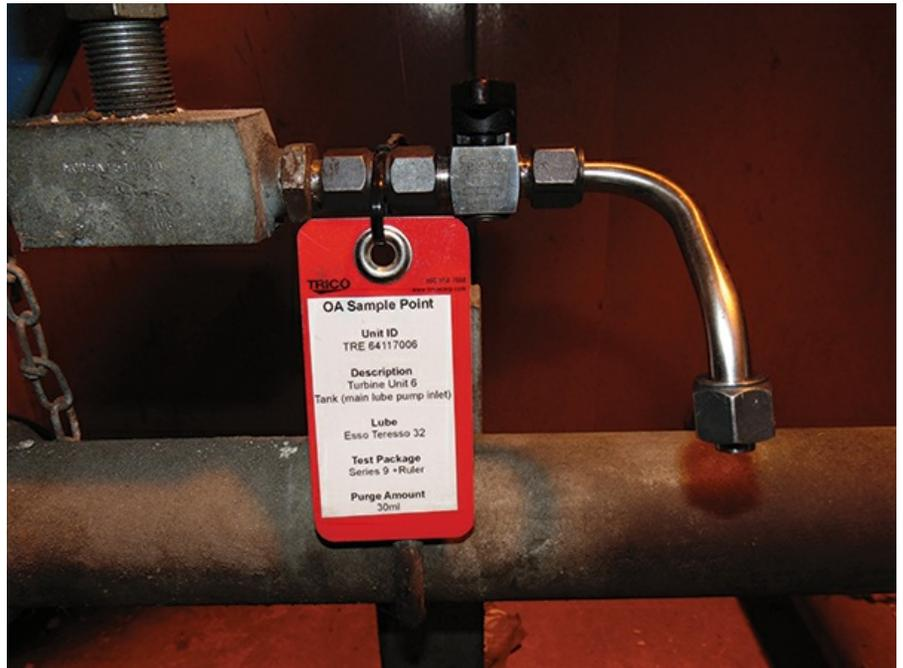
considered a measure of the performance of the lubrication tasks. Viscosity or mismatched additives can be an early indication of cross contamination of lubricants. Alternatively, lagging performance indicators, such as the acidity of the lubricant, signs of wear, or progressing failures, signify existing problems.
